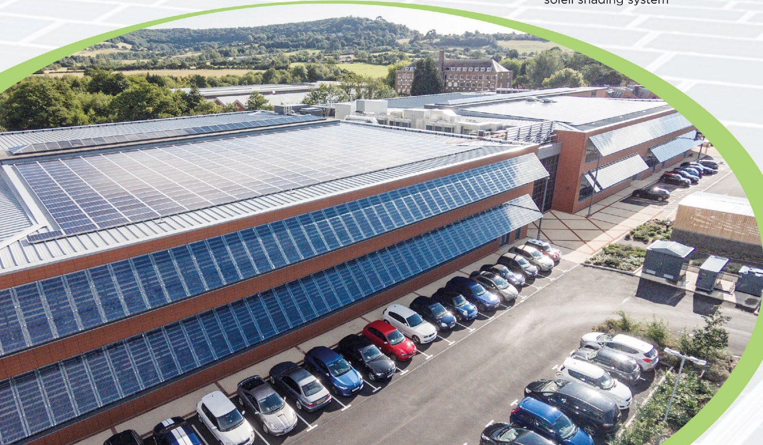
IMAGE (BELOW): Renishaw Innovation Centre 241.25 kWp solar PV system & 49.89 kWp bespoke solar brise soleil shading system
