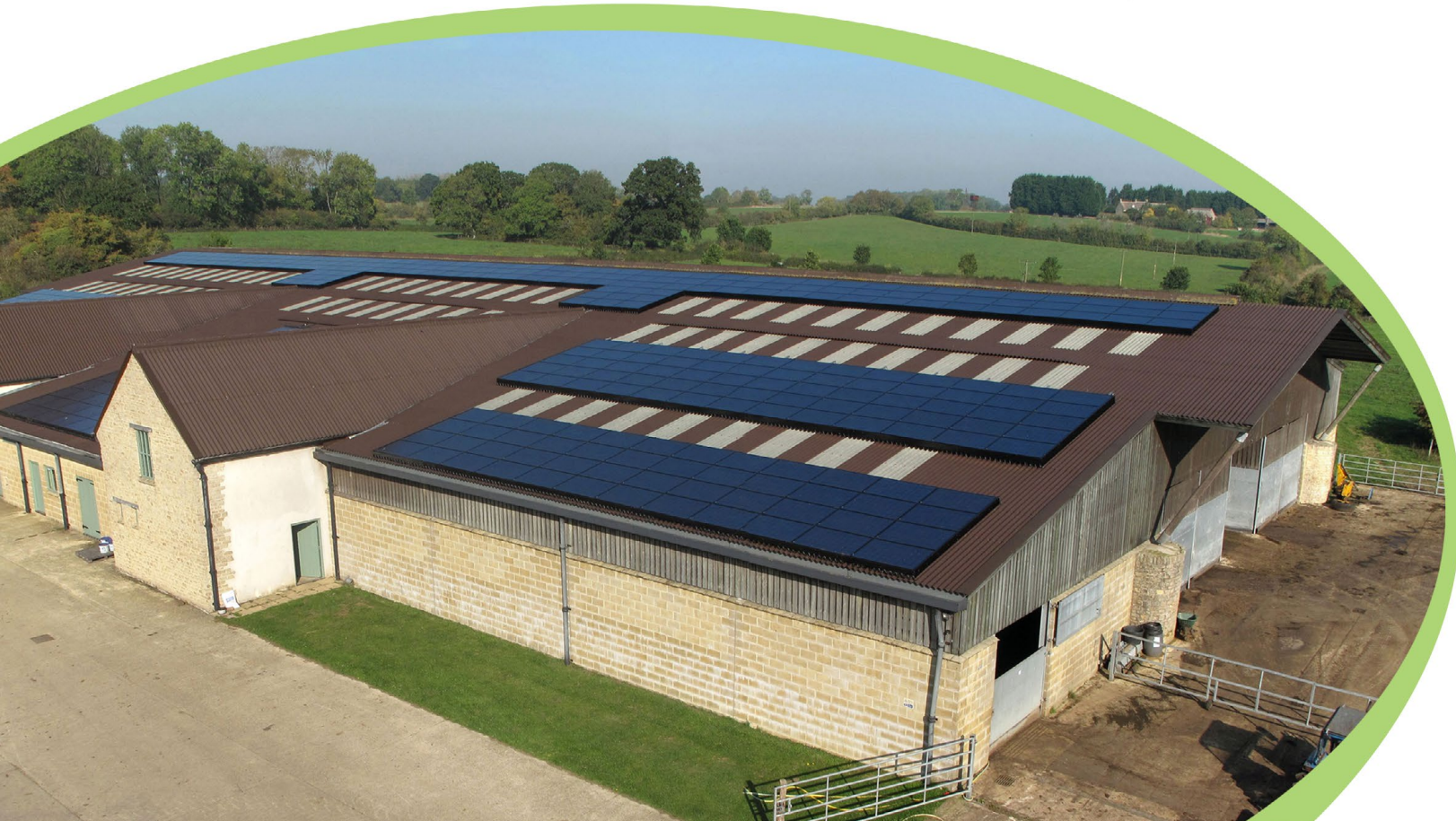
IMAGE (BELOW): Duchy of Cornwall Estate 99.64 kWp bespoke solar PV system One of six Solarsense installations Estimated annual output: 86,695 kWh Actual annual output: 98,850 kWh
