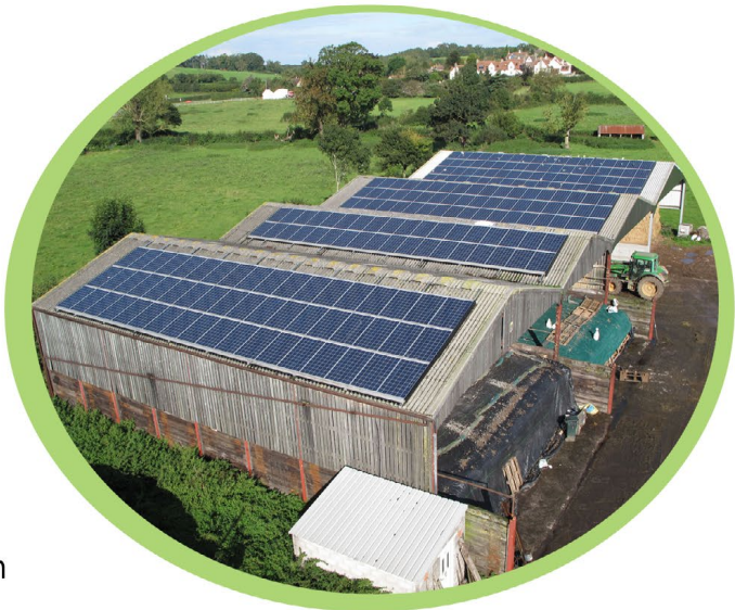
IMAGE (ABOVE): Varley Farm 50 kWp standard solar PV system Metal corrugated roof Delivering 10% more than predicted
